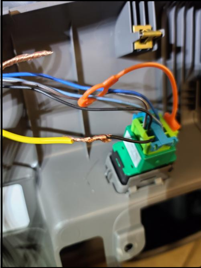
7. Yellow relay wire to Black on switch side
